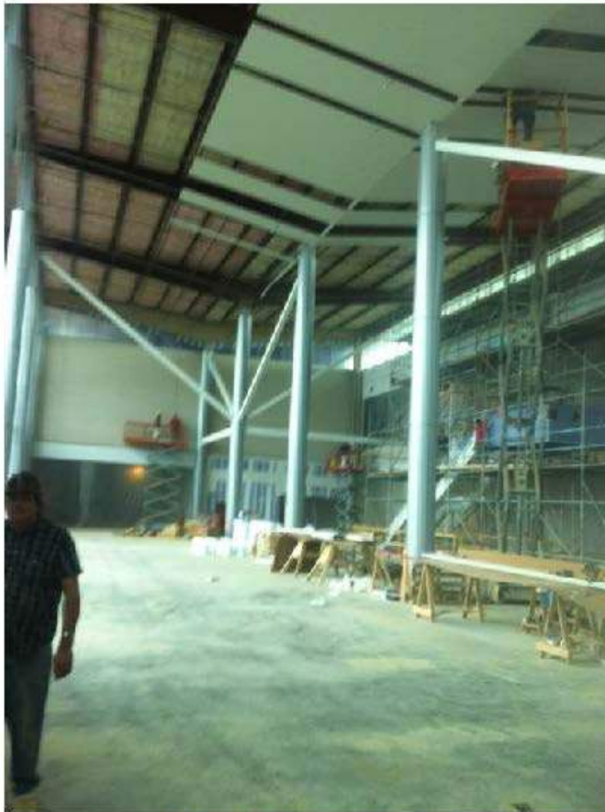
Looking into the two-story Reading Room.
