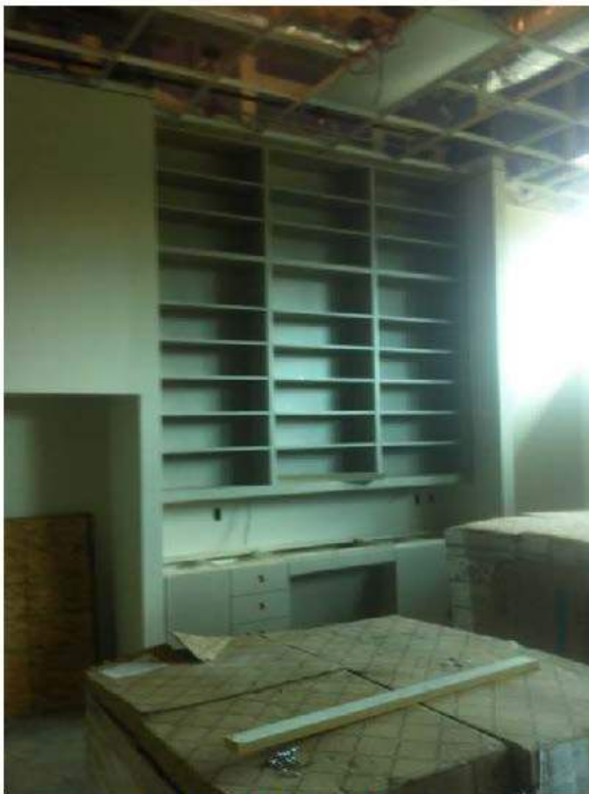
Looking toward the millwork in the Delivery Room.
