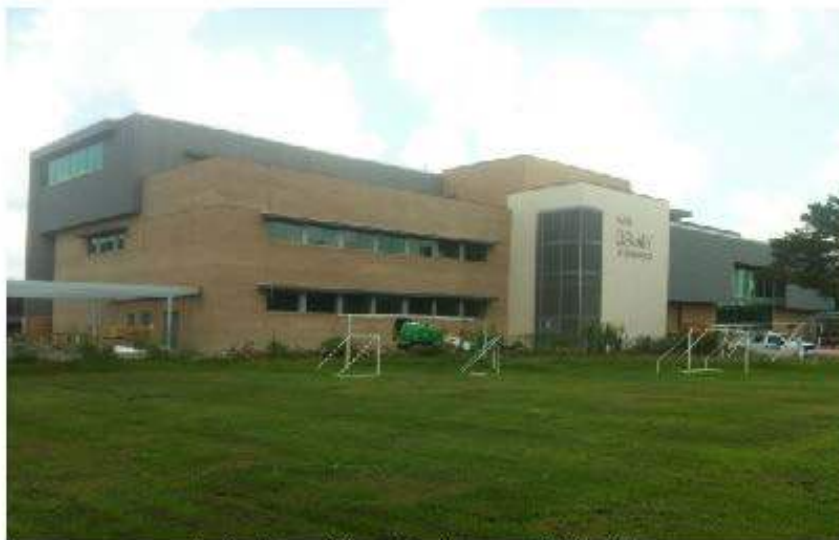
Looking toward the southwest corner of the building.
