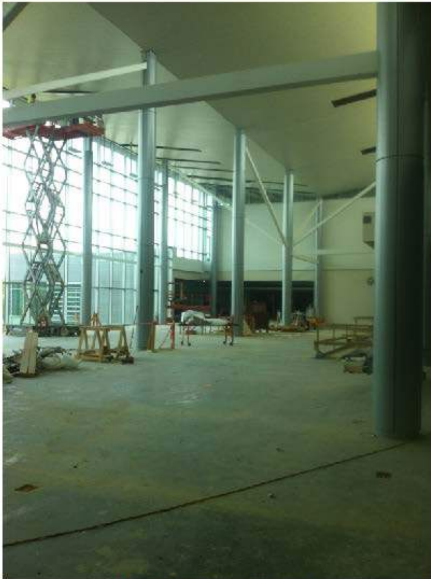
Looking east in the two-story Reading Room.
