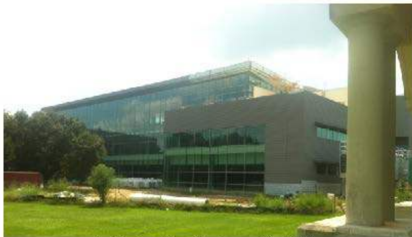
Looking toward the northwest corner of the building.
