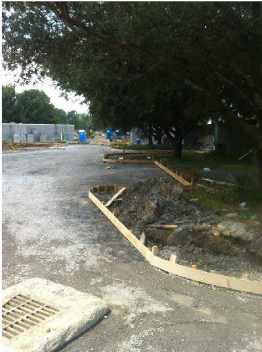
Looking west toward the Service Yard entry.
