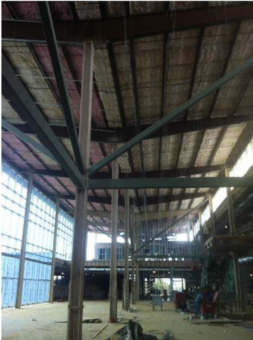
Looking at the underside of the "butterfly" roof.
