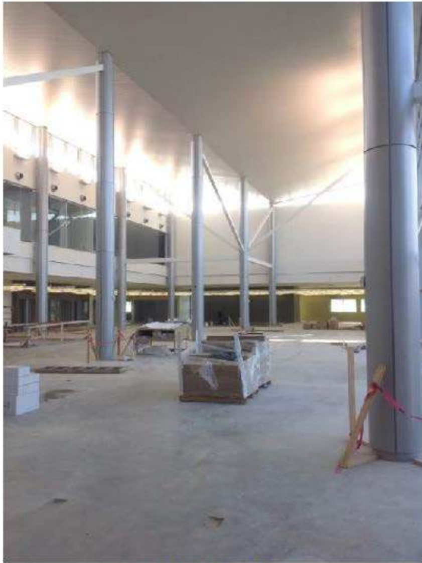
Looking west in the two-story reading room.
