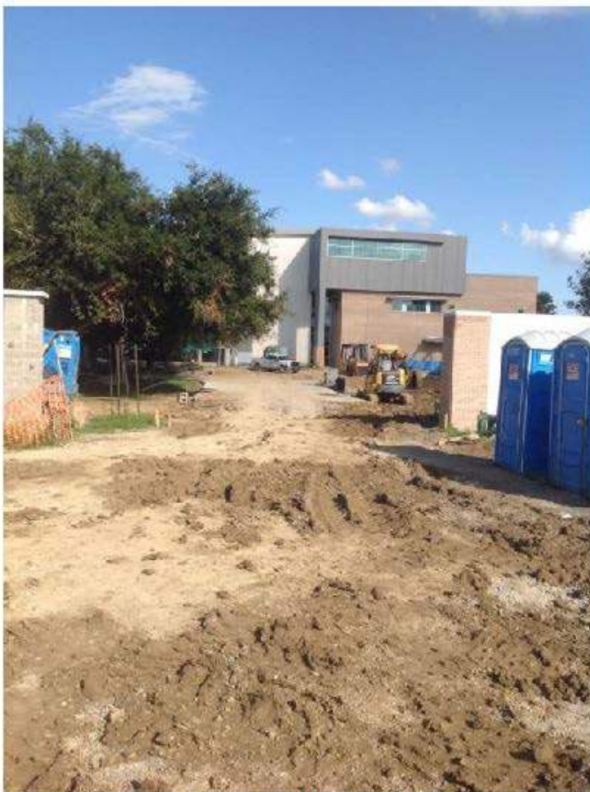
Looking east toward the Service Yard.
