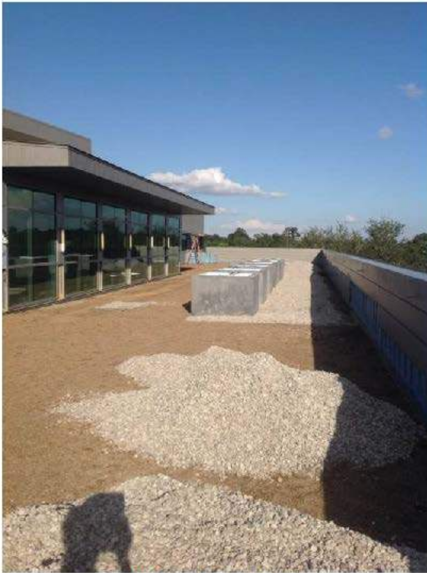
Looking east on the south vegetated roof.
