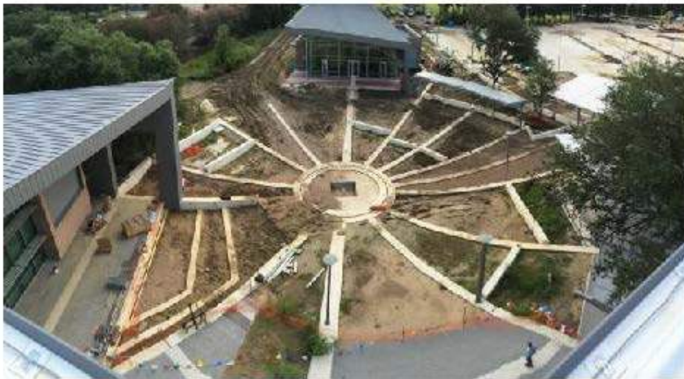
Looking from the roof to the Plaza.
