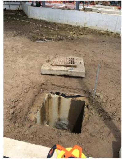
This catch basin is being lowered to ensure proper drainage.
