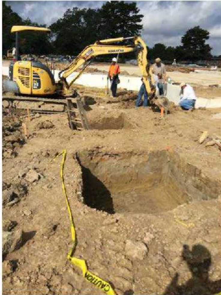
The flag pole foundations are being dug.
