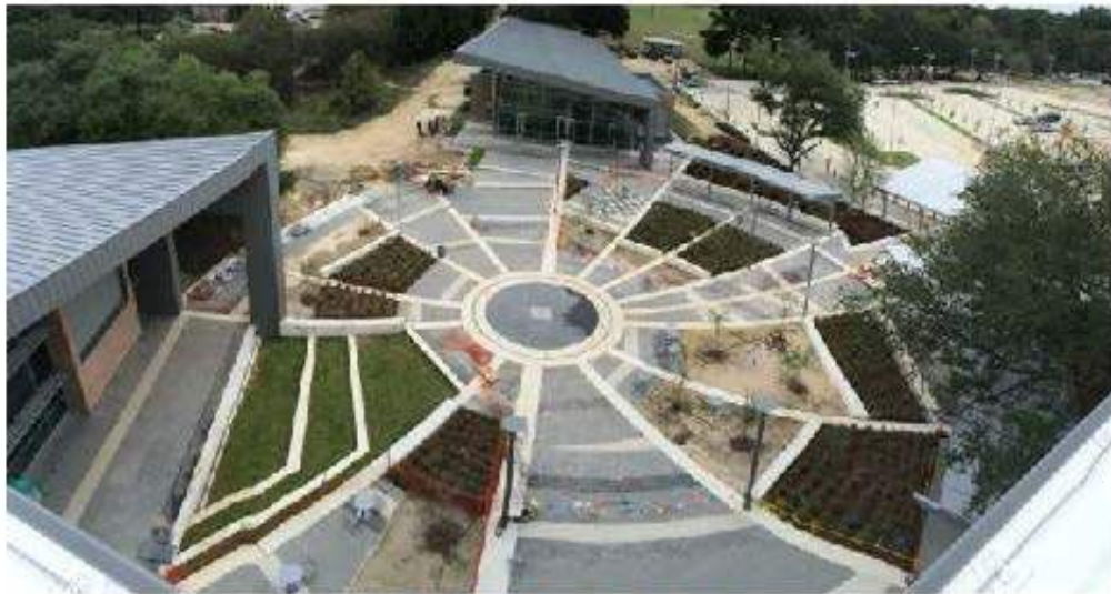
Looking from the roof to the Plaza.
