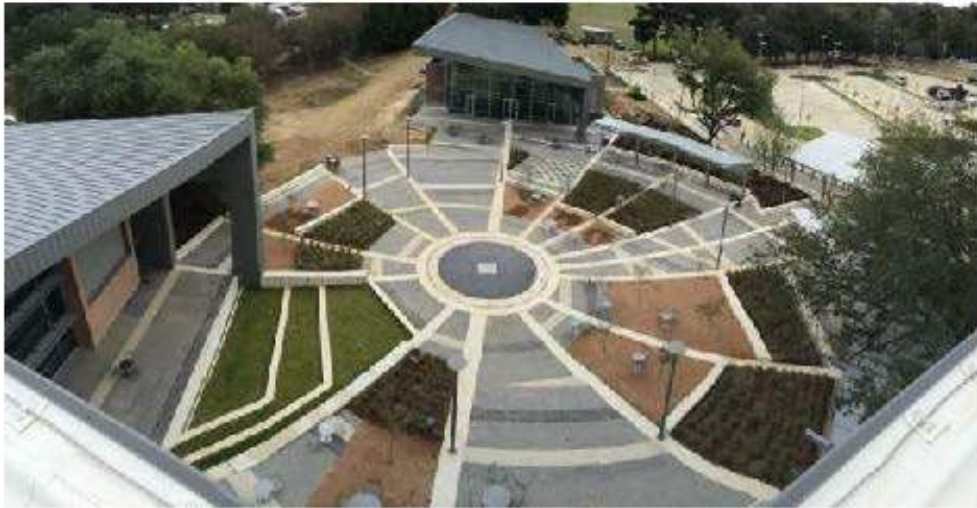
Looking from the roof to the Plaza.
