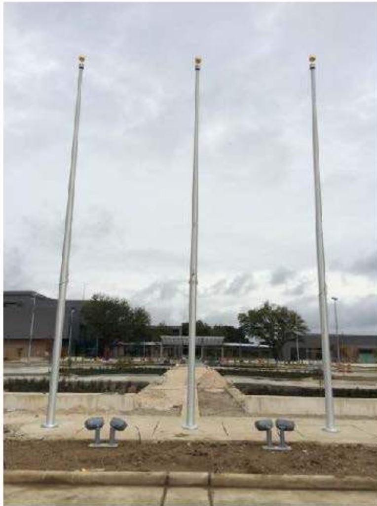
Looking from the parking lot to the Drop Off Canopy and the Plaza.
