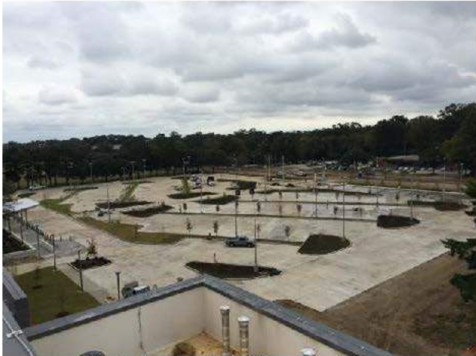
Looking from the southern roof garden to the new Goodwood parking area.
