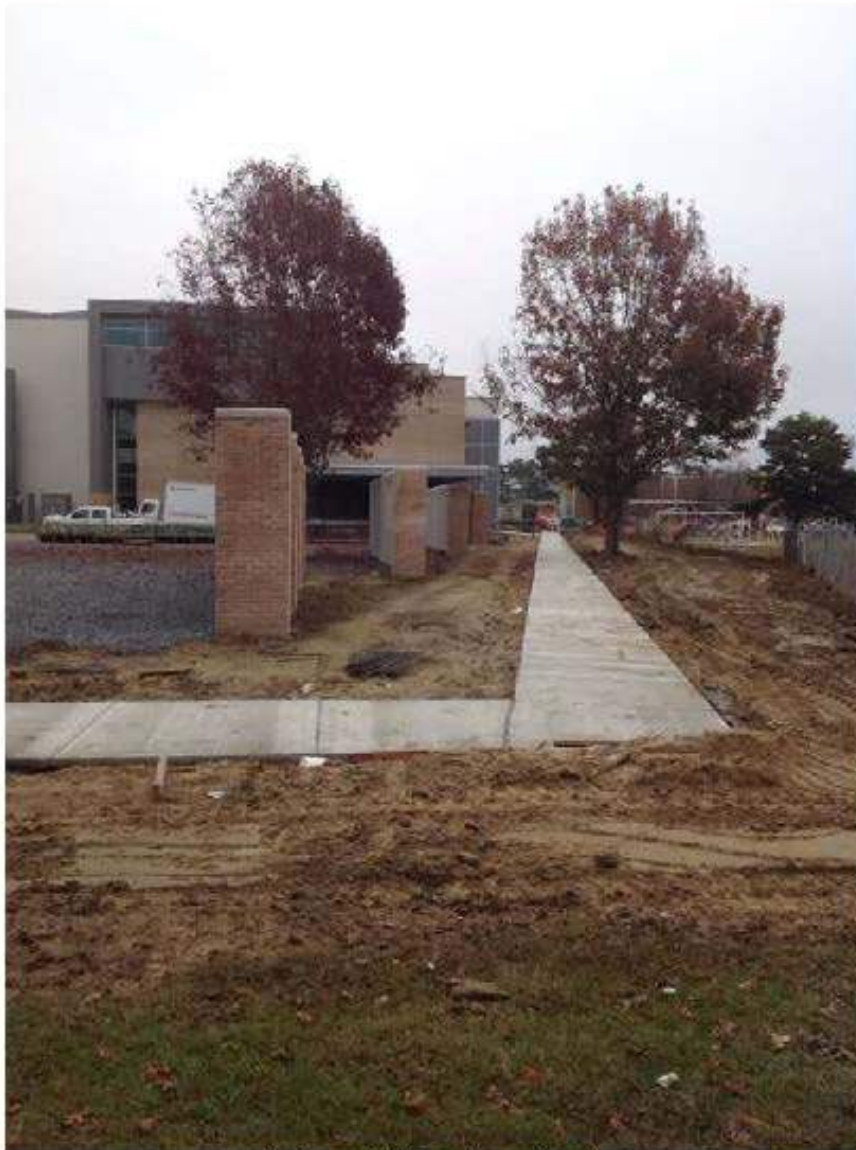
Looking east at the southern sidewalk.
