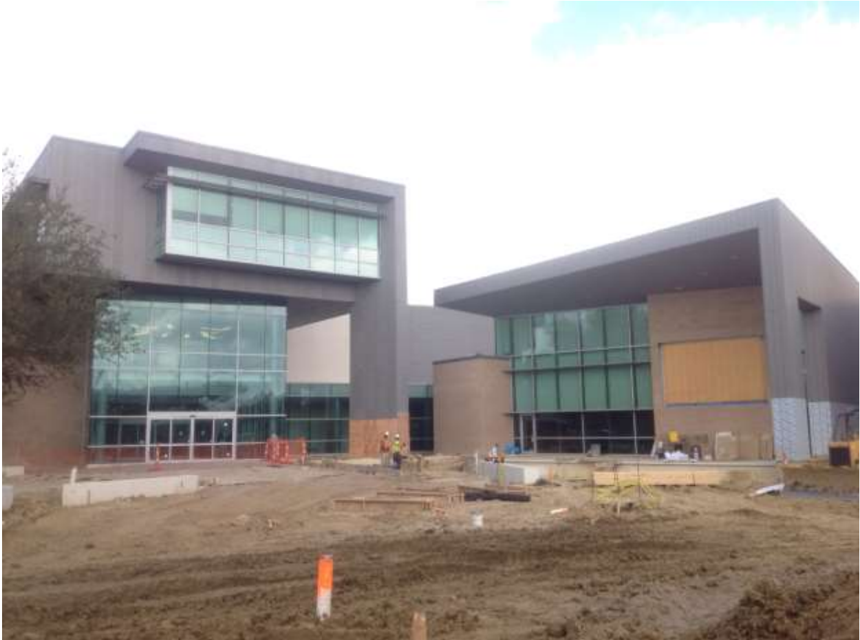
Looking toward the Library entry.
