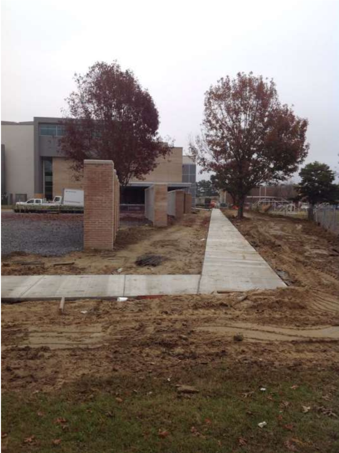
Looking east at the southern sidewalk.
