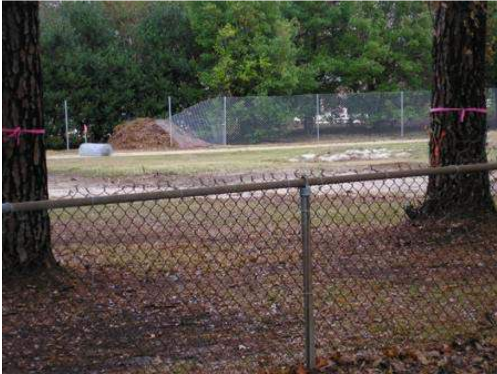
Installation of Construction Site Fencing 110911
