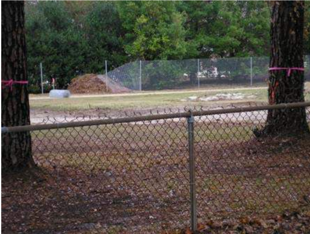
Installation of Construction Site Fencing 110911
