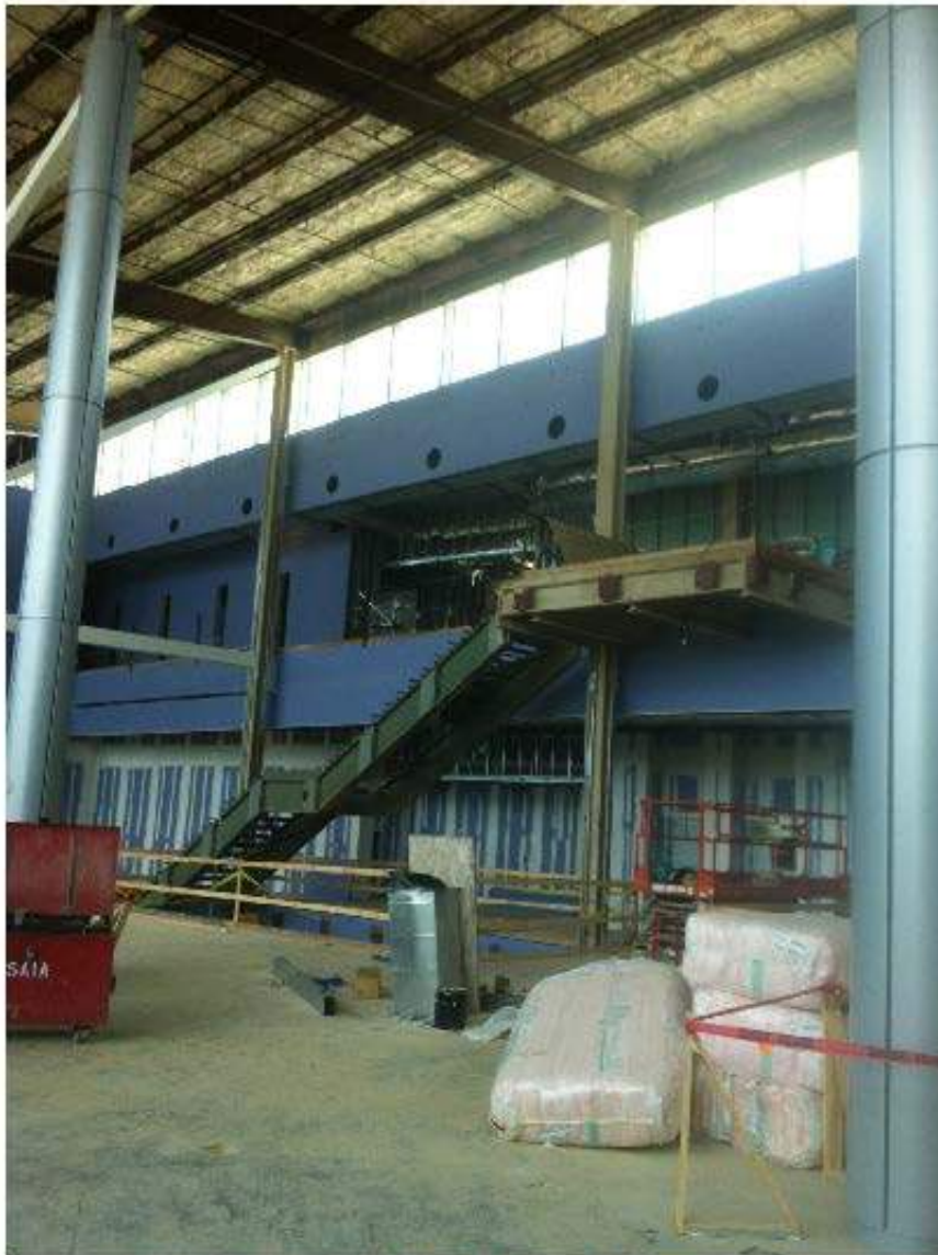
Looking toward the monumental stair in the two-story Reading Room.
