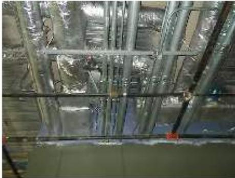
Access to VAV Box 8-7 blocked by electrical conduit.
