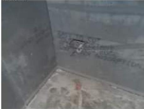
Copper water line not insulated as required.
