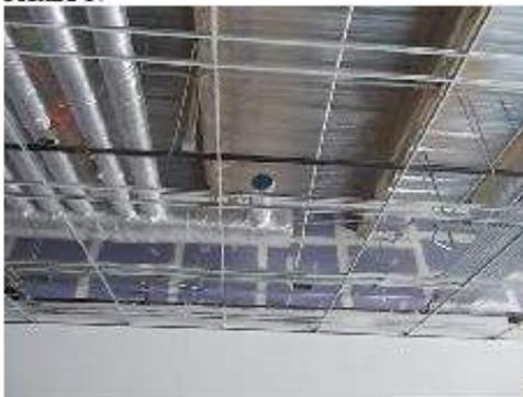
Hole punched in plastic cover on duct end.
