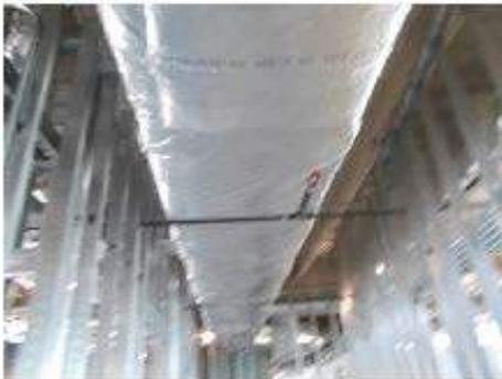
Sprinkler pipe compressing duct insulation.
