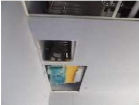
Fan Coil Unit at 3<sup>rd</sup> level stair No. 3 not fully protected.
