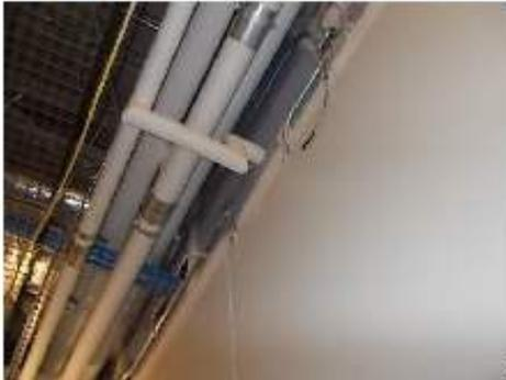
Pipe insulation is not continuous through wall penetration
