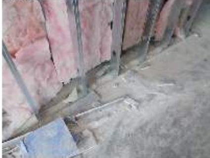
Clean construction dust, dirt and debris from wall cavity prior to installing sheet rock. Numerous location throughout 3<sup>rd</sup> floor.
