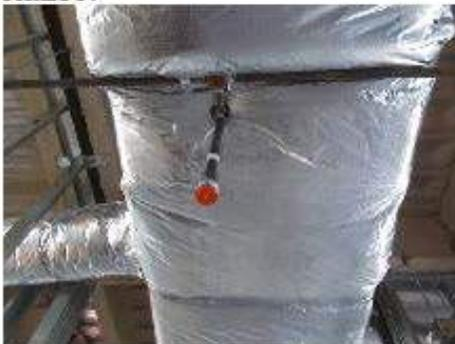
Sprinkler pipe compressing duct insulation.
