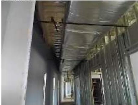
Sprinkler piping compresses duct insulation at numerous locations throughout.
