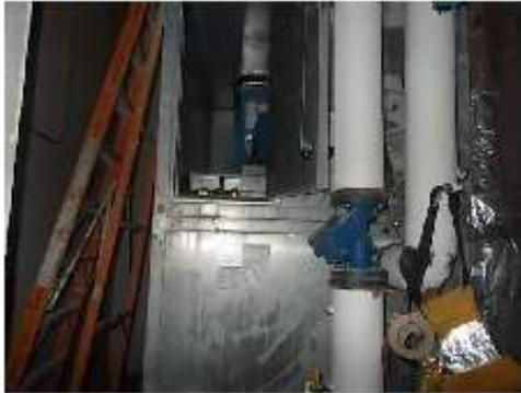
Protect inside of AHU when not working on unit
