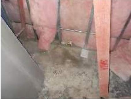
Trash in wall cavity with sheet rock being installed.
