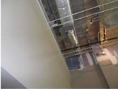
Verify sufficient access to controls on VAV Box 3-8
