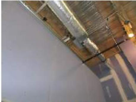
Verify easy access to VAV box. Box not labeled in field. (Possibly Box No. 3-8 on plans)
