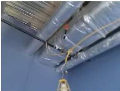
Separate sprinkler line from duct and reinsulate as needed. Provide sufficient space for duct insulation.
