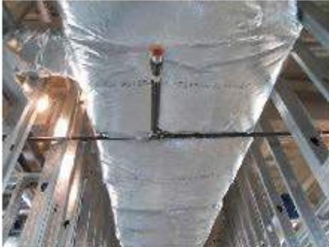
Sprinkler pipe compressing duct insulation.
