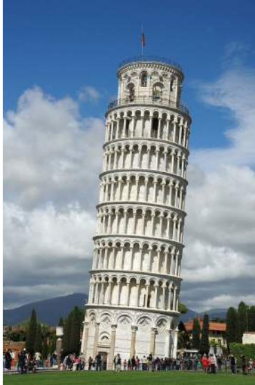
Leaning Tower of Pisa, Italy
