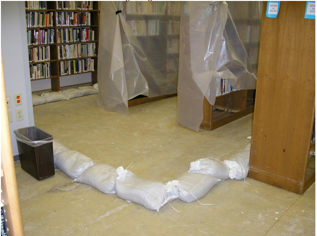
Sand Bags in 600s to Contain Possible Water Intrusion 9/12/08
